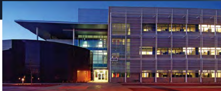
Sandia MESA Facility
